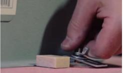
9. Clean silicone squeeze-out from around the cutout edges with your finger. Remove the masking tape and clean away any silicone that may have leached underneath. Wipe the edges with alcohol.
